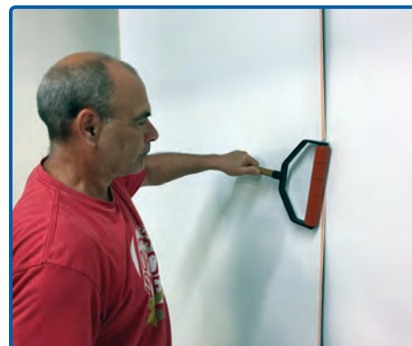
Use Everhard's lightweight wall roller with the 5" wood handle for up-close work.
